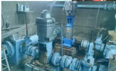
Vertical turbine replacement retrofit before and after.
