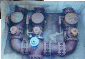
Glycol pump station valve vault rehabilitation before and after.
